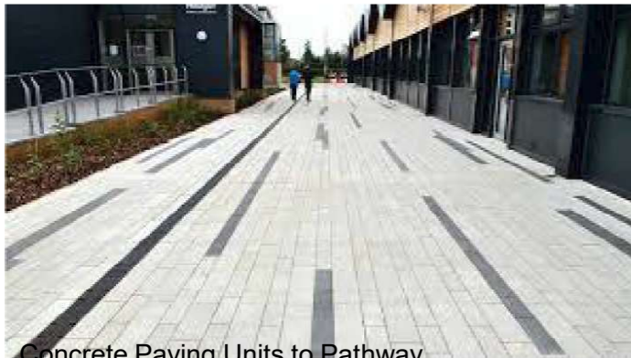
Concrete Paving Units to Pathway
