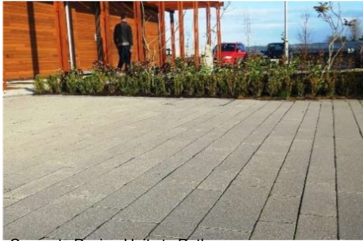
Concrete Paving Units to Pathway
