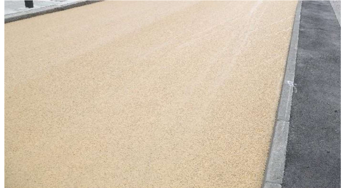
Buff Coloured Asphalt- Shared Surface between Plaza and LUAS
